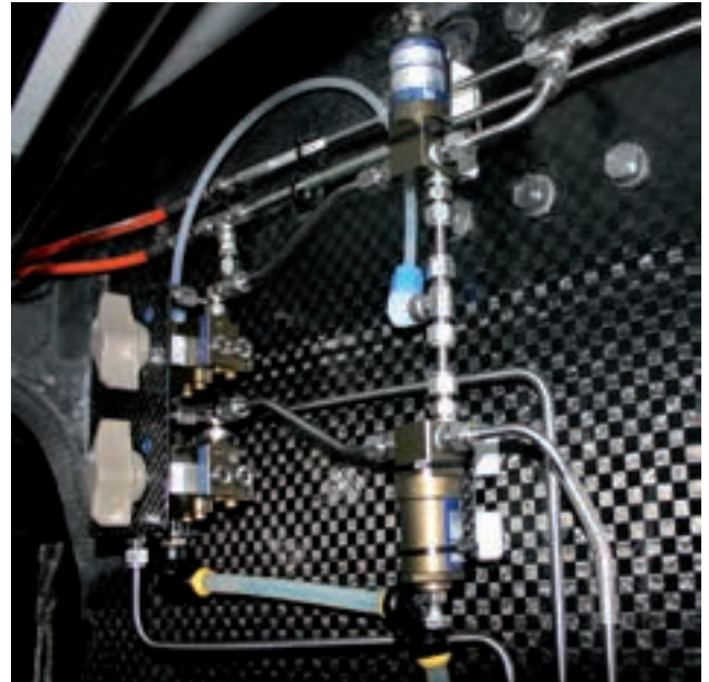
Installation of in-line valves
